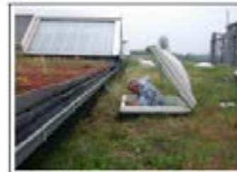
Example of green roof
